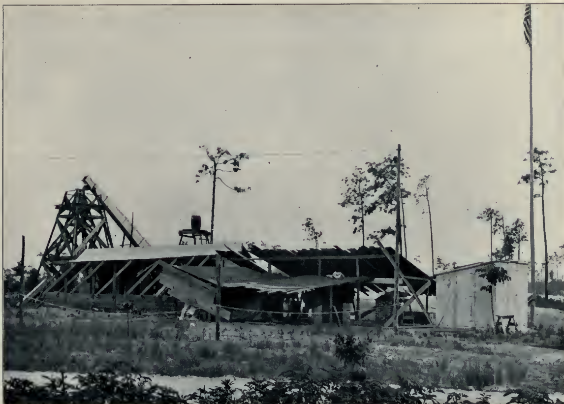
THE ECLIPSE STATION AT PINEHURST, N. C., LOOKING SOUTHWEST. Photographed by A. L. Colton.
