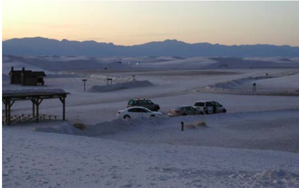
Figure 12. Dunes Drive. The National Park Service “plows” Dunes Drive in order to make the dune field more accessible to visitors. Because eolian processes constantly erode and transport the gypsum sand, continuous maintenance is required. Plowing the road has lowered the land surface in the vicinity of Dunes Drive, resulting in flooding and road closures during wet periods. Photograph by Katie KellerLynn (Colorado State University).
