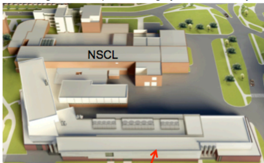
Existing National Superconducting Cyclotron Laboratory
