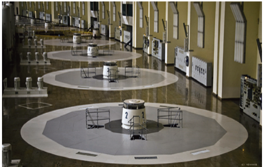
Figure 1. Sayano-Shushenskaya powerhouse machine hall operating floor prior to accident.
