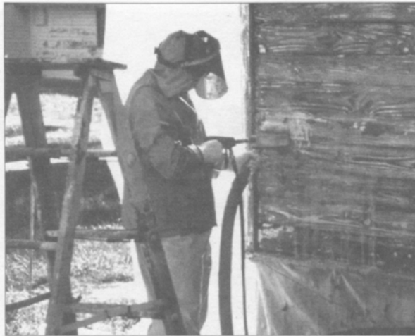
Environmental hazards of lead paint disposal can be reduced with engineered abrasives... and so can project costs.
