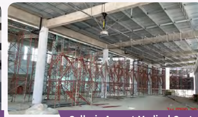
Galleria Area at Medical Centre
