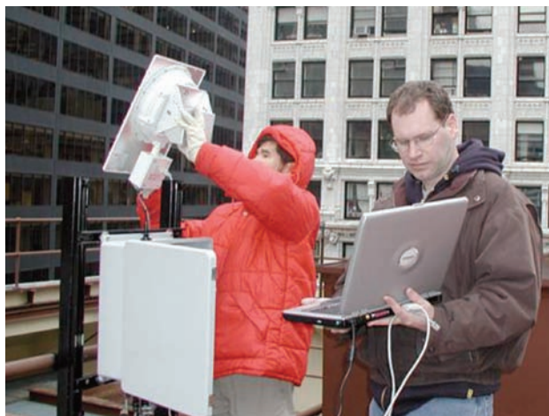
Installing and testing a networked sensor on a New York City building that will provide real-time data to emergency responders.
