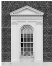
FIGURE 1 Windows are character-defining features in every historic public building. Stone quoins, Ionic pilasters and carved pediments frame multi-light, arched windows defining this Georgian revival facade. (Carol M. Highsmith Photography, Inc./GSA)
