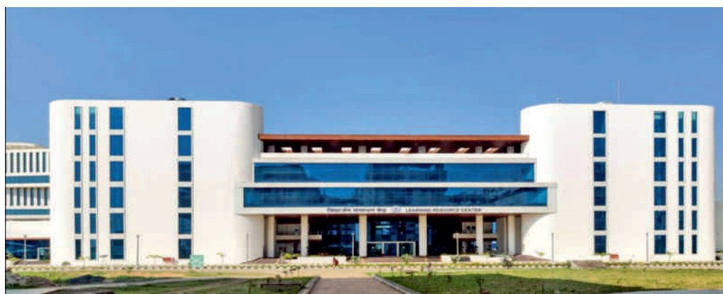
Figure 1. The Learning Resource Center (LRC) Building
