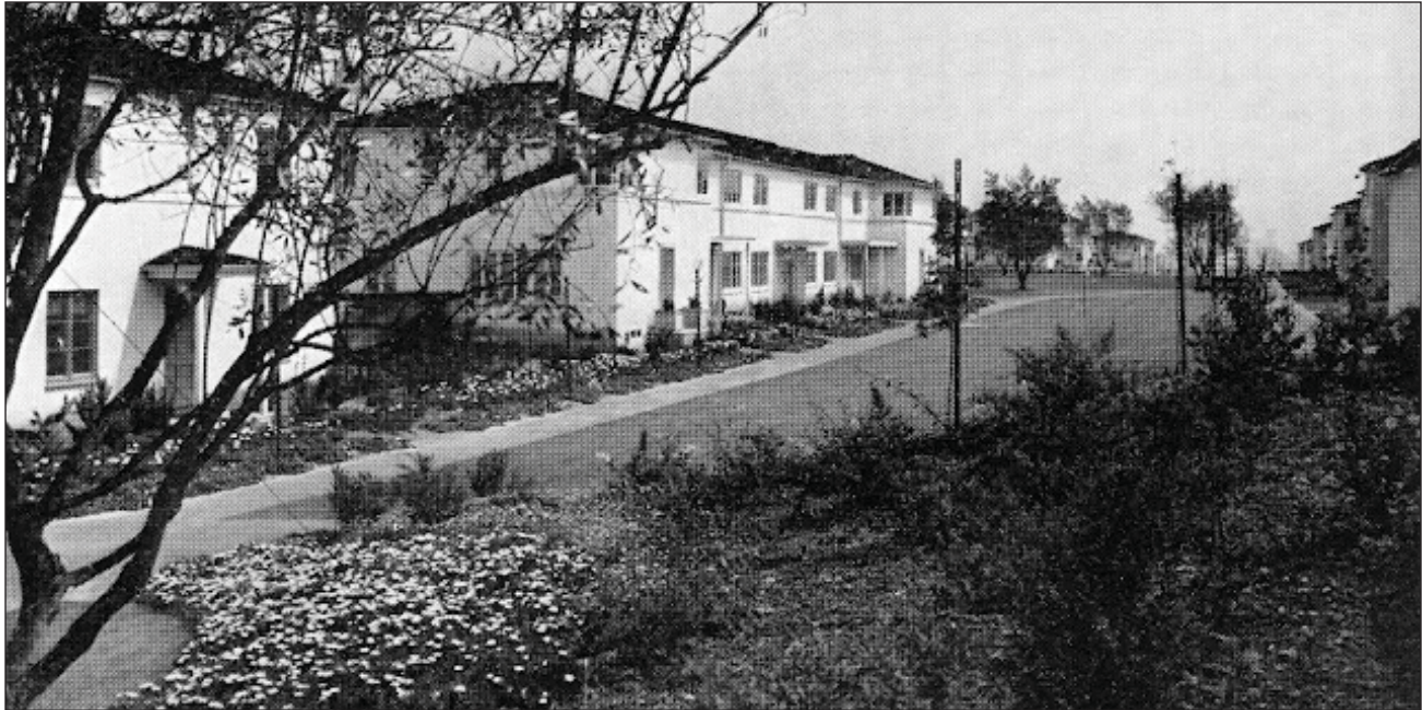
Wyvernwood, the first garden apartment in Los Angeles, c. 1940 (from Architectural Forum , May 1940)
