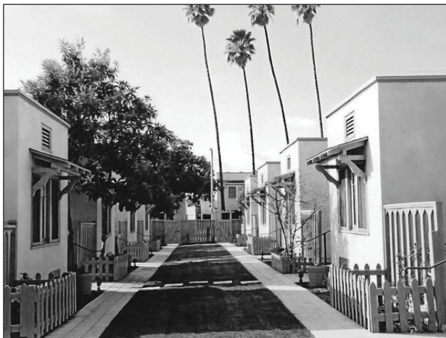
A typical 1920s bungalow court in Los Angeles ( Los Angeles Times , 2010)
