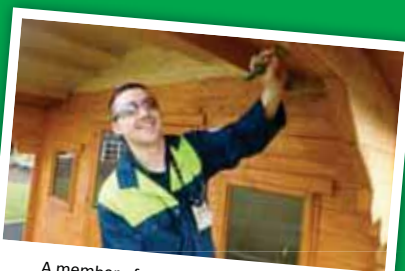
A member of staff from NIS Ltd (Chorley) painting the outdoor classroom with a protective woodstain.
