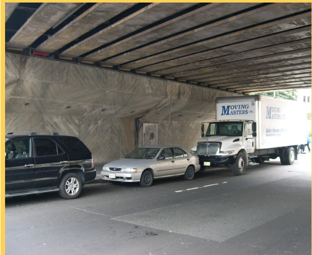
Figure B-3. Illegally Parked Truck Under Overpass
