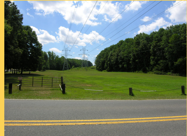
Figure 2-23. Utility Corridor Near Bowie
