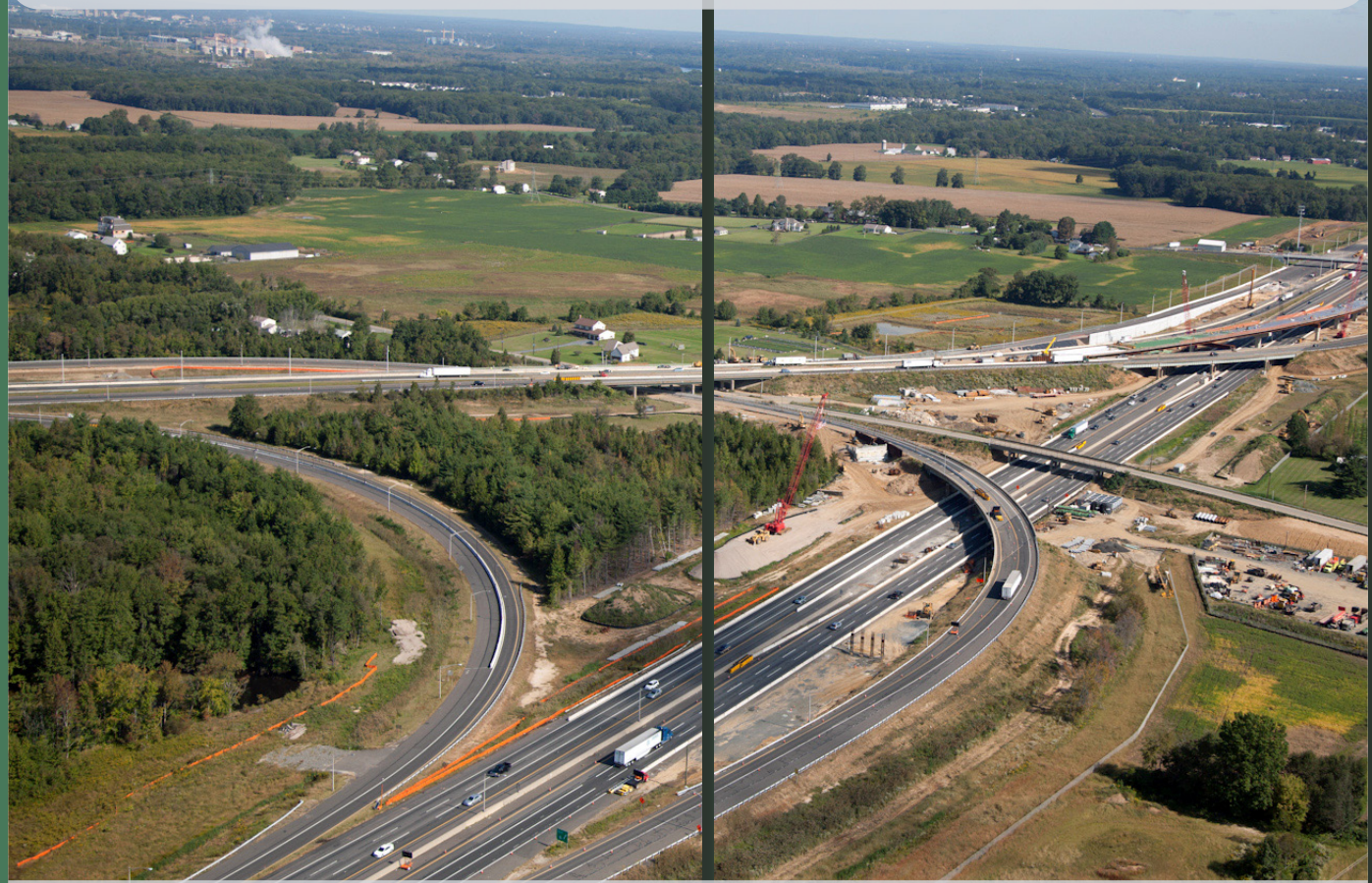
Turnpike Widening - Connection to Pearl Harbor Memorial Turnpike Extension
