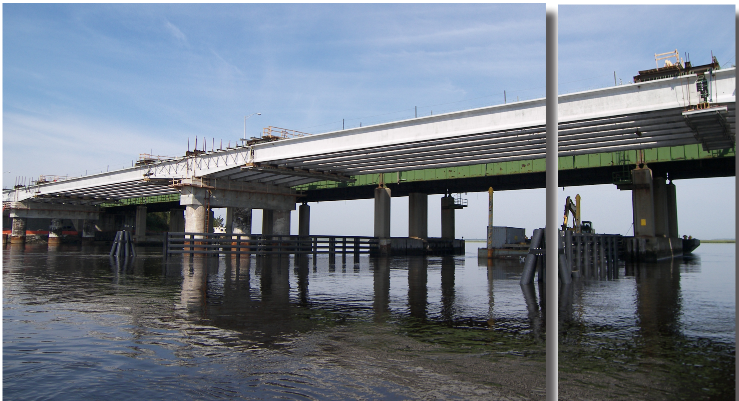
Parkway Widening - Mullica River Bridge
