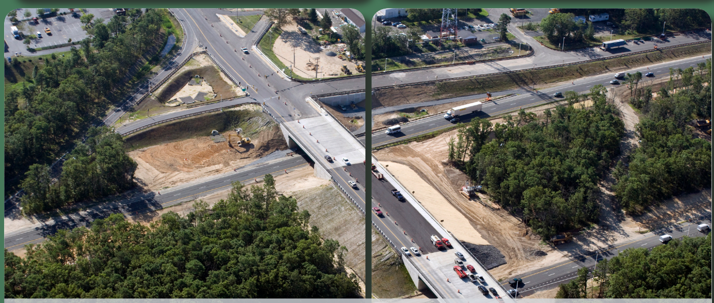
Parkway Widening - Improvements at Interchange 67
