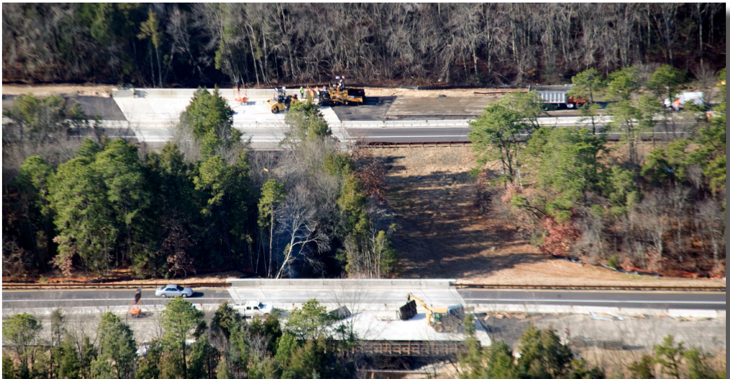
Garden State Parkway Widening - Bridge over Jake's Branch
