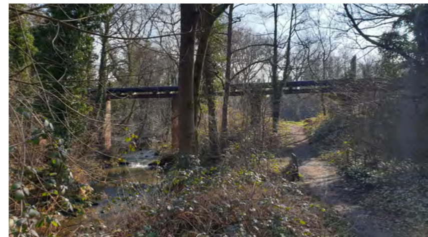
3 - Riverside walkway in Coronation Park and pipe crossing Leadmill Beck
