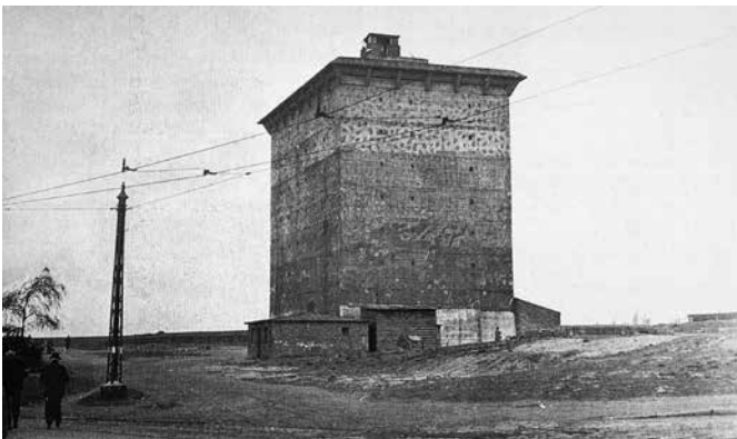
Hochbunker Kuniberg 1945 (National Archive Washington)
