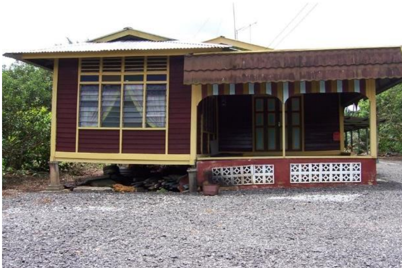
Fig. 8 Typical low-weight wooden building located in Johor, Malaysia
