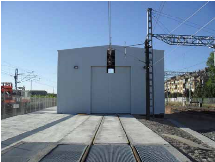
Albacete automatic track gauge changeover for trains
