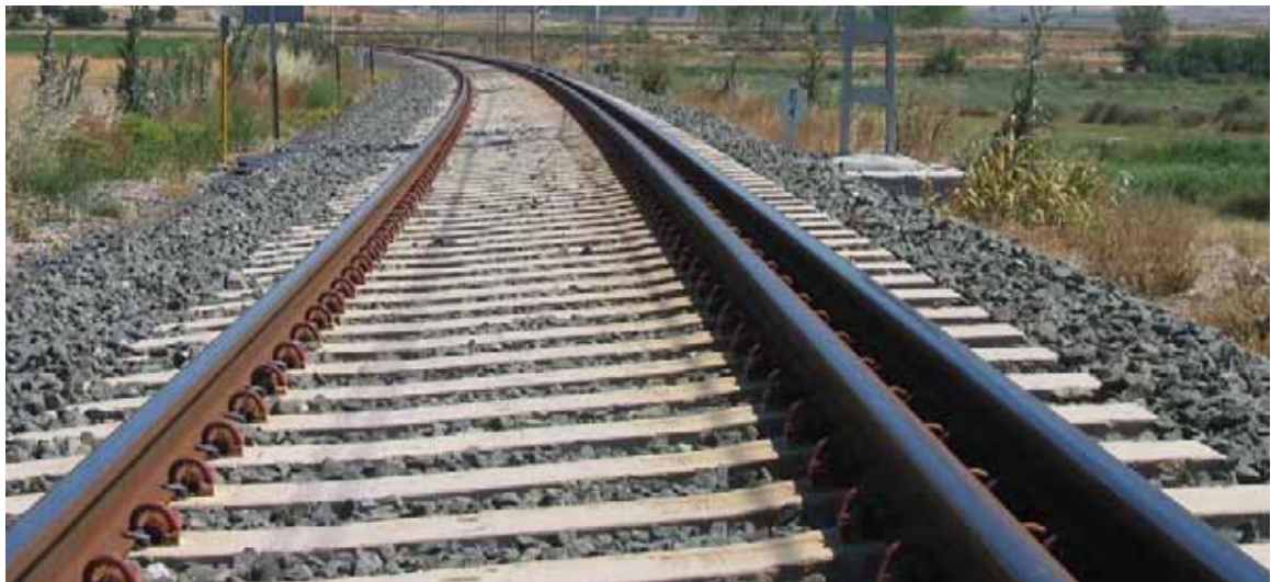
Three-rail track that allows the running of trains with two track gauges (in this case, Iberian and standard)
