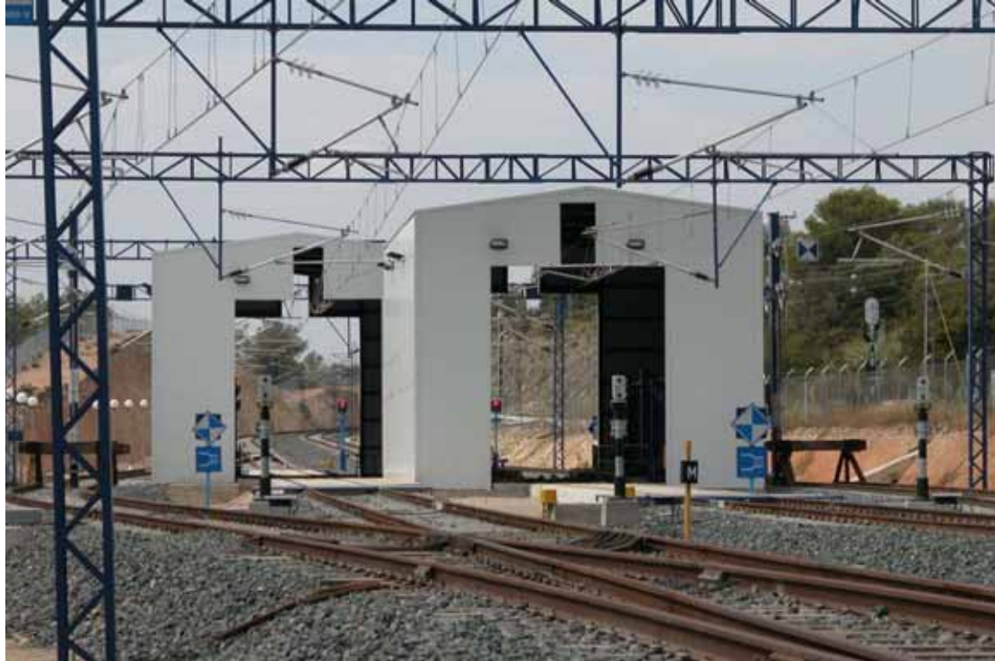
The double changers at Roda de Bará (in the photo) and Antequera allow trains that run in opposite directions to change gauge simultaneously
