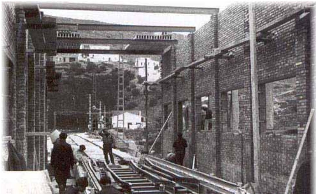
Construction of the Portbou changer (Photo: Francisco Uriz)
